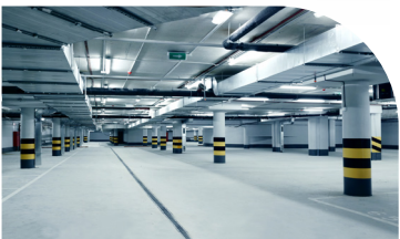
ENCLOSED CAR PARK
